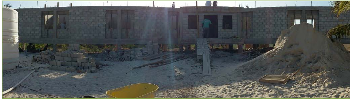
Initial phase of Staff and Visitor Quarters, May 20, 2015
