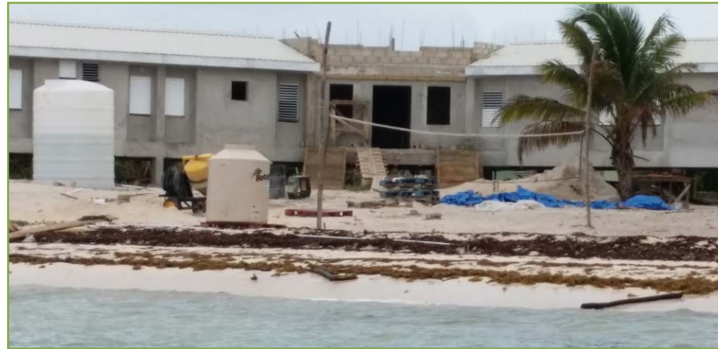
Initial phase of Staff and Visitor Quarters
